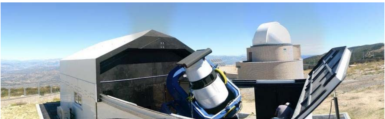
Fig.7. Astronomical Observatory of Montsec at Pre-Pyrenees Mountains, 1570m MSL height. Foreground, the TFRM inside its reinforced glass-fiber enclosure, with its sliding roof opened and the South wall end lowering.
