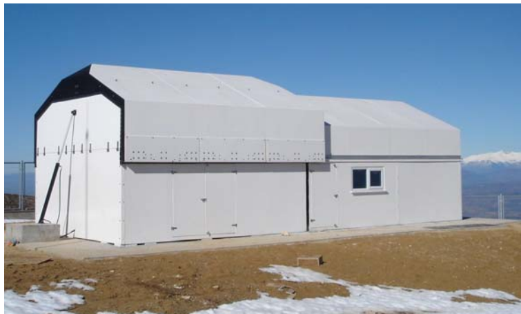
Fig.4. Reinforced glass-fiber enclosure designed and constructed by GRPro, Inc. Note the North-South sliding roof and the South downloadable end wall which allows observing at low altitudes.
