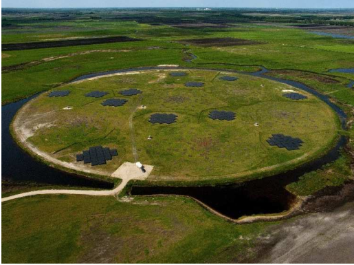
Figure 1: Photograph of the LOFAR superterp – pictured are twelve HBA core fields (grey squares) and six LBA fields (barely visible).
