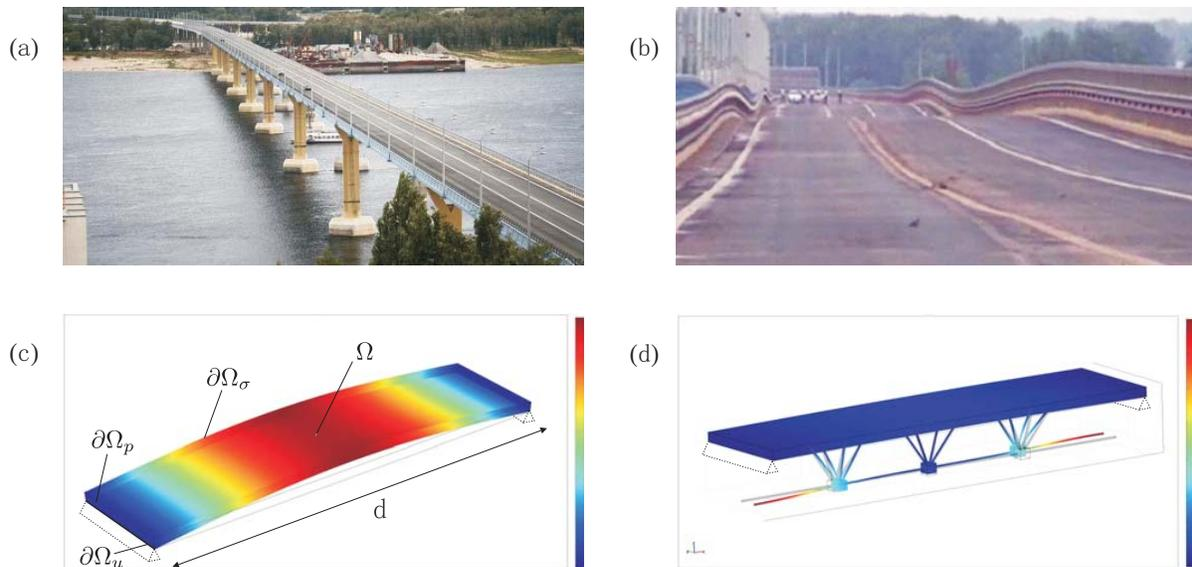
Figure 1: Volga bridge, ((A), (B) HTB Volgograd News). Flexural deformation of the main upper body of the bridge: (B) real structure, (C) simplified numerical model, (D) modified 3D structured wave guide with lightweight resonators.
