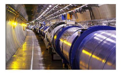
Figure 10. The LHC tunnel with its accelerating magnets.
