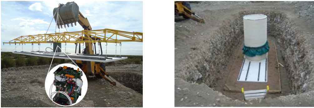
Figure 8. (lhs) First module buried at the Observatory site, the insert shows the electronics inside its enclosure; (rhs) Muon counter placed over sand bed with service pipe installed, about to be buried.
