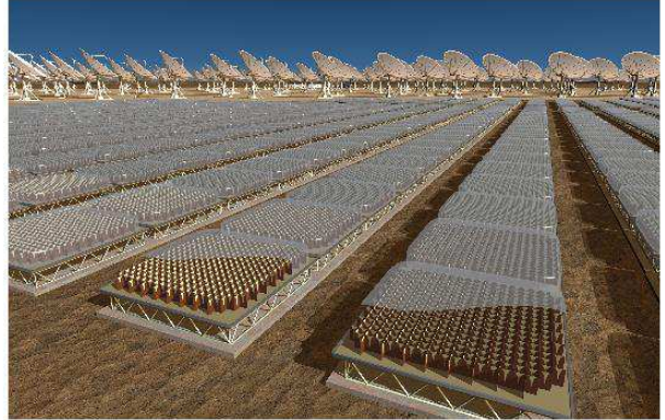
Fig. 2. SKA reference design: aperture array for low frequencies and parabolic dishes for high frequencies (Copyright: SKA Programme Development Office and XILOSTUDIOS).
