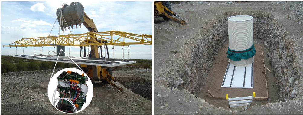
**FIGURE 6.** (left) First module buried at the Observatory site, the insert shows the electronics inside its enclosure; (right) module in the well placed over a sand bed with service pipe installed, about to be buried.
