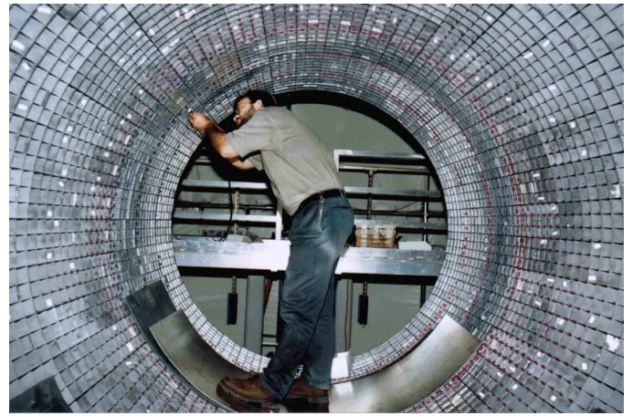
Fig. 5. Photograph of the inside of the barrel calorimeter during construction.
