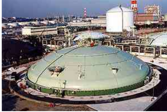
Figure 10: Photograph of cryogenic storage tank of volumes \approx 200,000 \text{ m}^3 .
