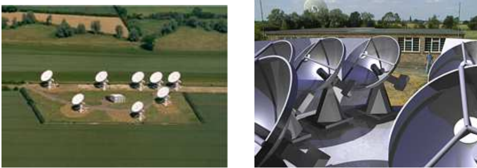
Figure 4. Artists impressions of the two arrays comprising AMI. (Left) the 13-m antennas of the Ryle Telescope, showing the planned change to a 2-d array. (Right) The array of 3.7-m antennas.
