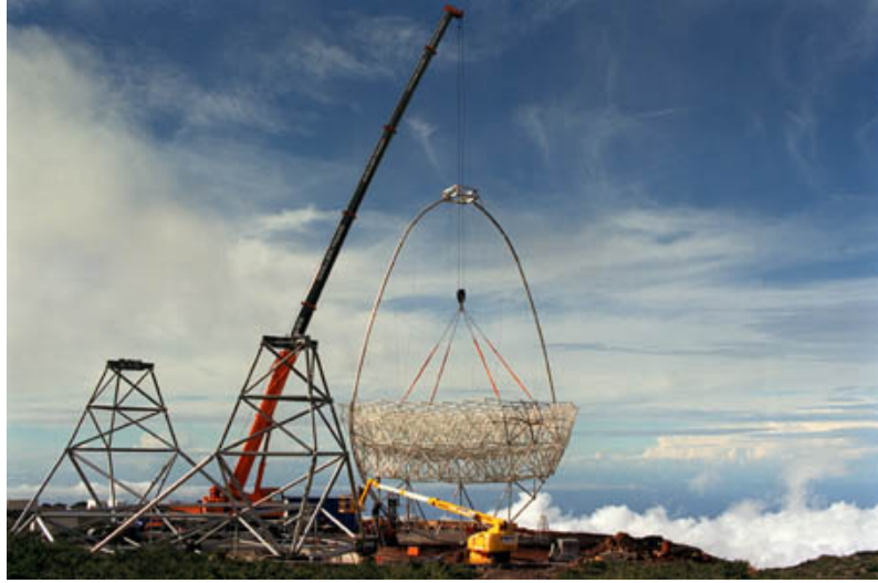
Fig. 1 Mirror and camera support structure of the MAGIC-I Telescope being positioned on top of the azimuth rail. Credit: R. Wagner.
