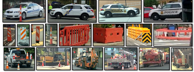
Figure 4. Variations and Challenges in Work Zone Objects. There exists a large variation in work zone objects and work vehicles in the ROADWork dataset and this difference is geographical in nature. For instance, police vehicles (first row) have different designs (dependent on locality) and the appearance of barriers, vertical panels or tubular markers (second row) varies across cities. Work vehicles (third row) show large variations as they are specialized to the kind of work being performed in the work zone.
