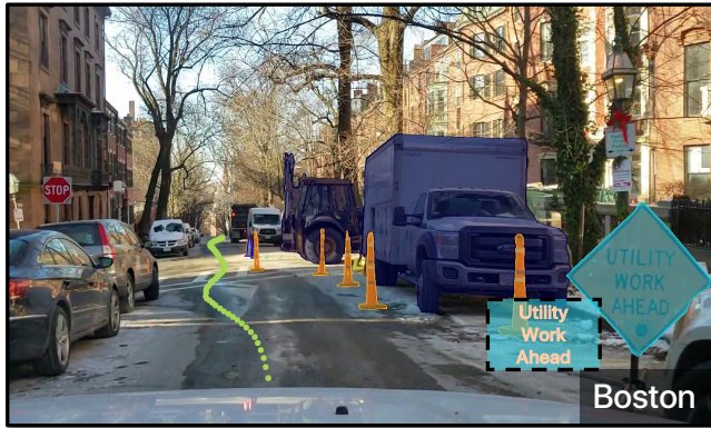
Tubular markers and cones next to work vehicles on right side of road.
