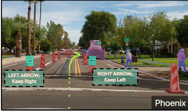
Work on corner next to road. Workers off road. Line of vertical panels on both sides of road lane. Work vehicle partially blocking road.
