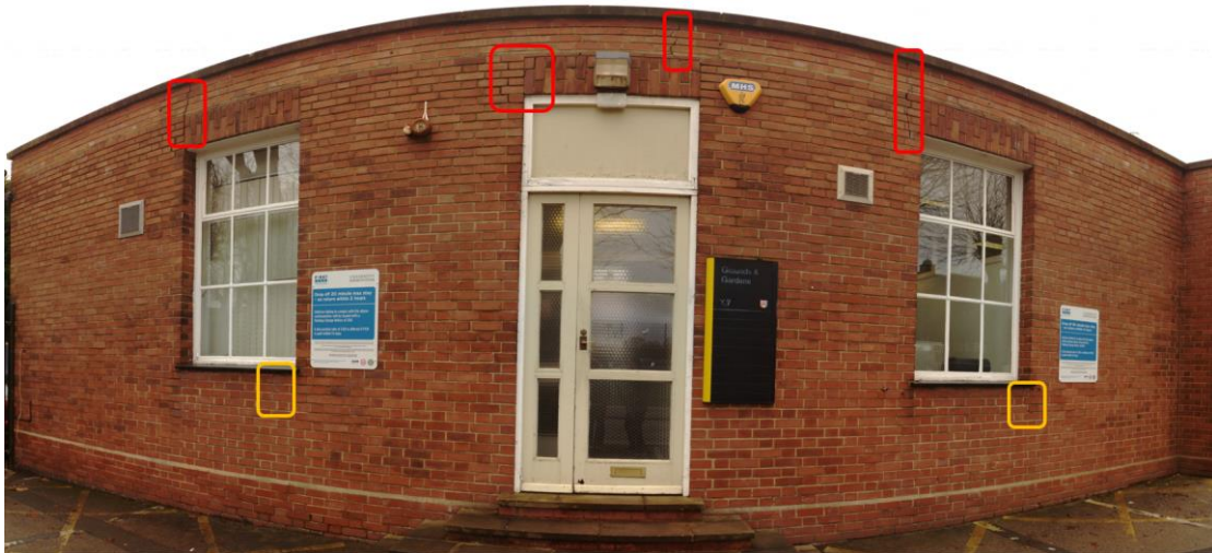
(b) Panoramic image of masonry wall.
