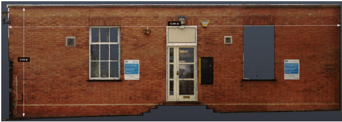
(a) Point cloud results of masonry wall.
