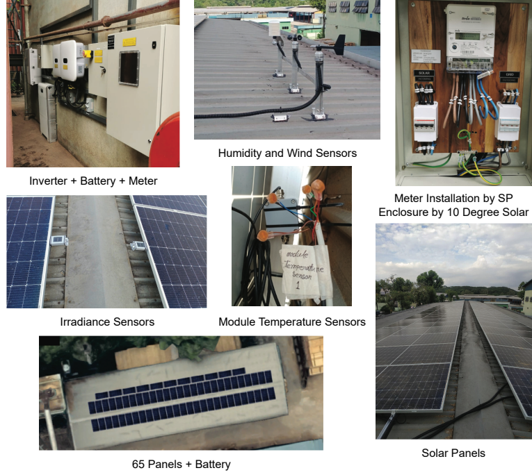
Figure 7: LHT Holdings Solar PV system.
