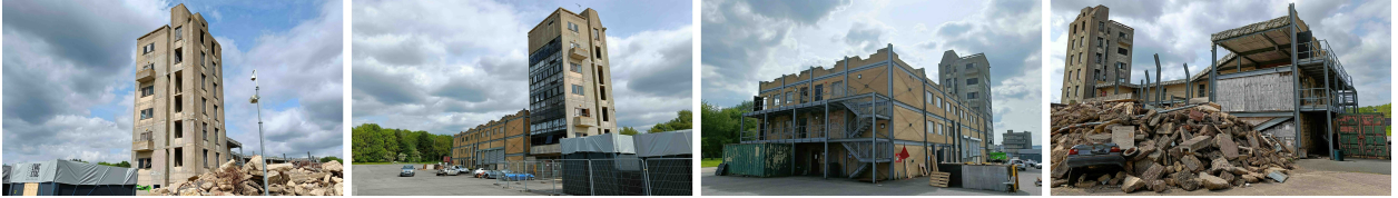
Figure 10: Photographs of the Rig 5 site. It is a large site, 52x29x27m (LxWxH) in size, which contains multiple structures and is staged as a disaster scenario. The site is comprised of a seven storey building next to a long three storey building with an exposed interior on one side and a metal fire escape at one end. There is a large rubble pile next to these buildings with several upright metal girders within it.
