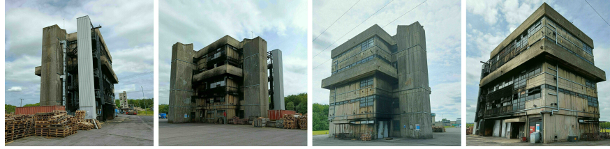
Figure 9: Photographs of the Industrial Building B site. It is a five storey building, 27x20x21m (LxWxH) in size, with a balcony surrounding the fourth storey and two concrete fire escapes attached to different sides of the building. There is also an exposed metal fire escape with a garbage chute attached to the building, which is comprised of thin metal structures and proved challenging to map.
