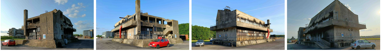
Figure 8: Photographs of the Industrial Building A site. It is a two storey building, 30x16x12m (LxWxH) in size, with a balcony surrounding the upper storey, which is partially enclosed on one side. There is a concrete fire escape on one corner of the building, a garbage chute (red) attached to one side, a concrete chimney and various metal structures on the roof.
