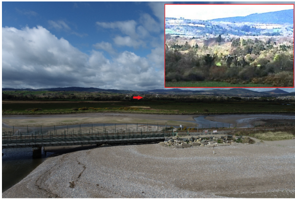
Fig. 15: Newcastle scenario: Two drones deployed to survey the railway bridge. The red arrow indicates the target drone in the image captured by the camera of the sentry drone (monitoring drone). The small picture inside the image is captured by the high resolution camera of photogrammetry drone.
