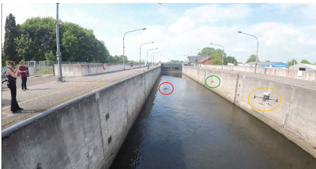
Fig. 17: Harburg Lock scenario: Two drones (circled red and green) deployed for an inspection survey, the third drone is (circled yellow) monitoring their separation distance.
