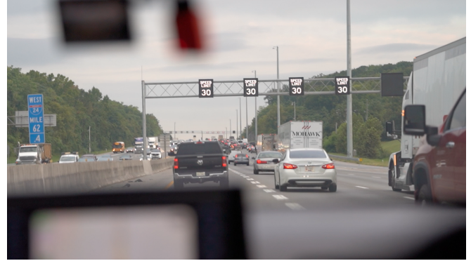
Fig. 1. Variable speed limit (VSL) system activated and posting 30 mph speed limit during congested traffic. Photo taken from the ego vehicle which automatically adjusts its velocity to 30 mph in response to the VSL system.
