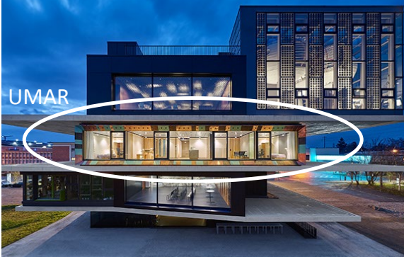
Figure 2: NEST building, Duebendorf, with the UMAR unit in white circle. © Zoey Braun, Stuttgart.
