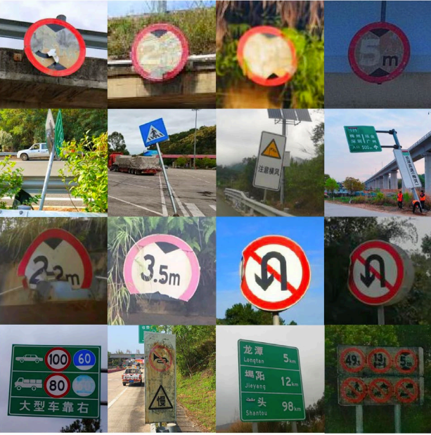
Figure. 1 Some of the damaged traffic signs in our dataset.
