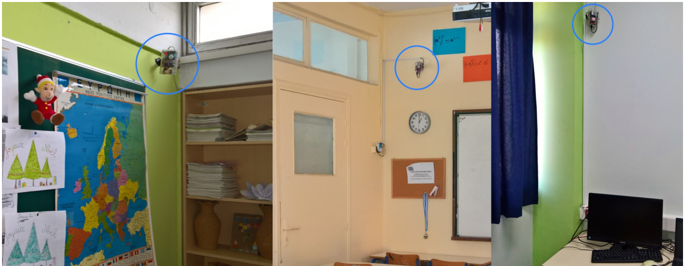
Fig. 2. Some examples of installations of the IoT nodes inside the school buildings participating in the GAIA project, with the IoT nodes circled to pinpoint their location. The nodes were installed above a certain height to prevent damage or accidents, as well as minimize acting as a visual distraction to students.
