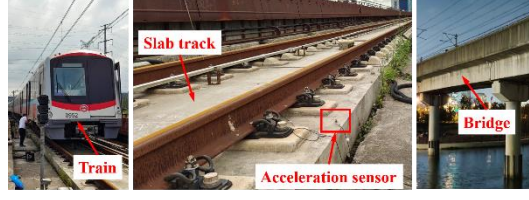
Fig. 8. Placement of acceleration sensors.
