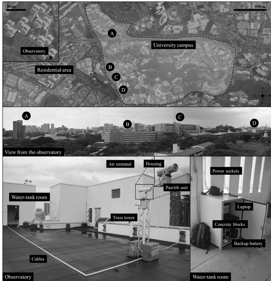
Figure 1: Observatory installed on the rooftop of the residential area in Singapore and its captured information. Source of the imagery: Google Earth. [15]
