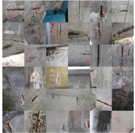
Figure 5: Input images of bridge rebar exposure
