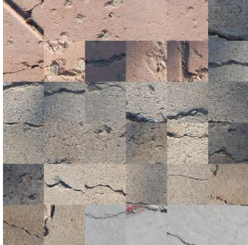
Figure 2: Input images of SDNET pavement crack
