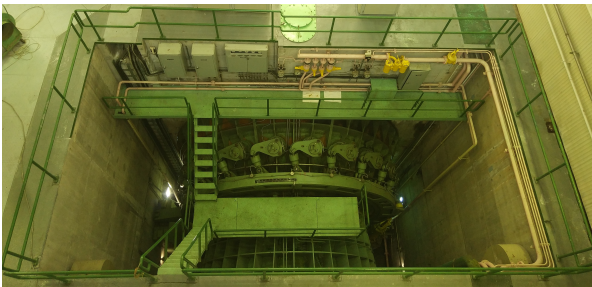
Fig. 5: PPC power generator for electricity production
