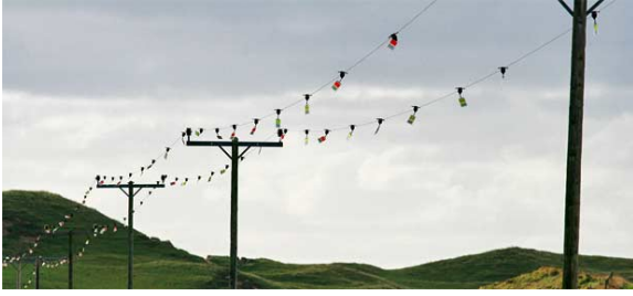
Figure 1: An example of bird diverters installed on a medium voltage power line infrastructure.
