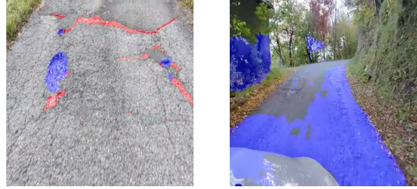
Figure 9: Two frames extracted from two different videos and used for qualitative evaluation of PUCP-MAnet predictions. On the left, we show an example of its very good performance on top-down videos. On the right, the issues in predicting road damage on wide-view videos.
