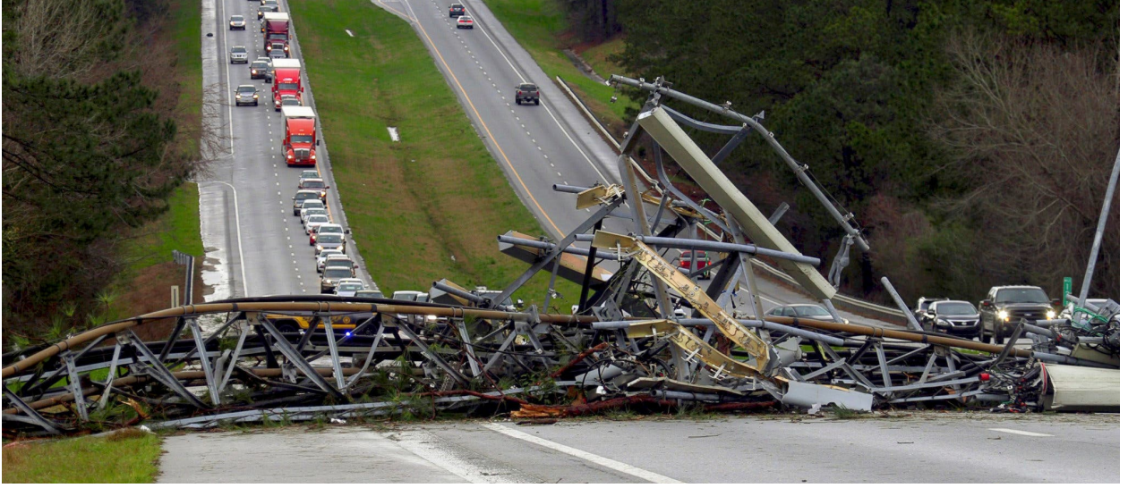
Fig. 1. Cell tower destroyed by a tornado [1].
