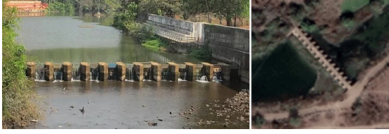
Figure 2: Photograph (left) and satellite image (right) of a gate based check-dam.
