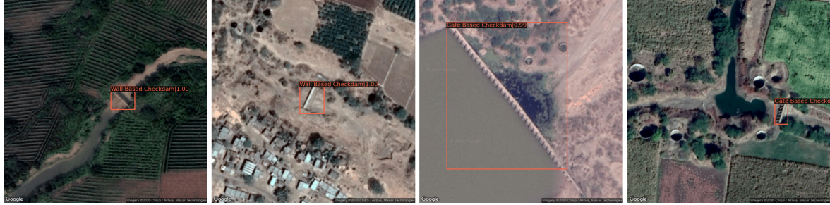
Figure 3: Object Detection results on the test data. (From left to right) a, b: Wall based check-dams detected among vegetation and dry surroundings; c,d: Detection on large size varieties of gate based check-dams.
