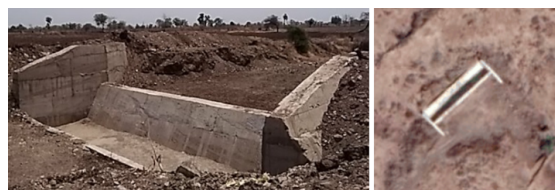
Figure 1: Photograph (left) and satellite image (right) of a wall based check-dam.
