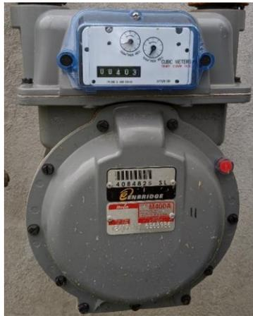
**Figure 1.** The Itron 400A gas diaphragm meter.
