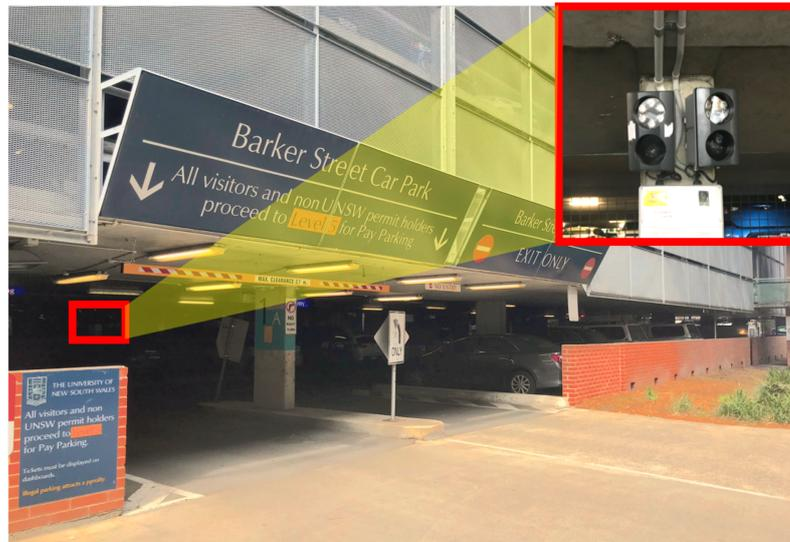
Figure 4.2: A real picture showing entrance and exit of our campus car park and a pair of LPR cameras installed side-by-side close to the ceiling of the car park ground floor.
