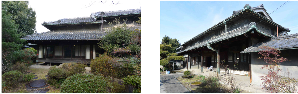
Figure 7: Exterior photos of house with pantile roofs.
