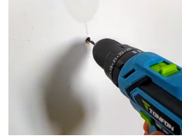
Figure 2: Drilling for sensor embedding.
