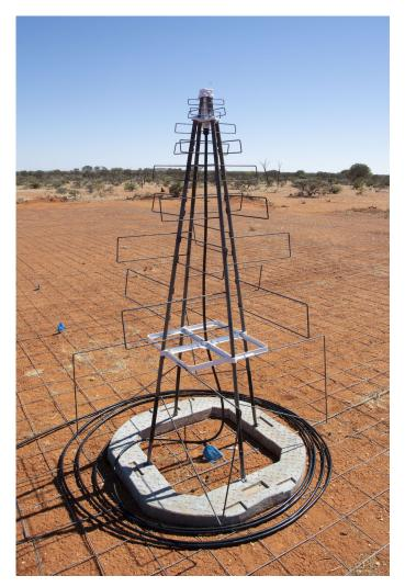
Fig. 3. SKALA2 antenna installed as part of AAVS1.
