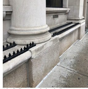
Alt: Spikes on a ledge in Boston to prevent sleeping or sitting.
