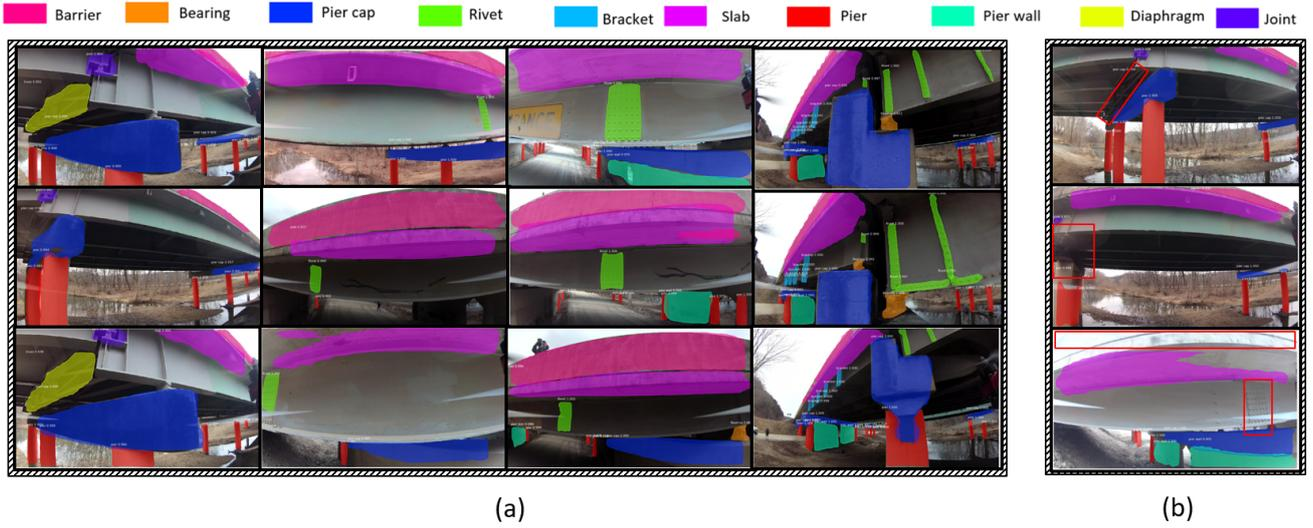
**Figure 8.** Examples of (a) successful detection and segmentation, and (b) false negative detection.
