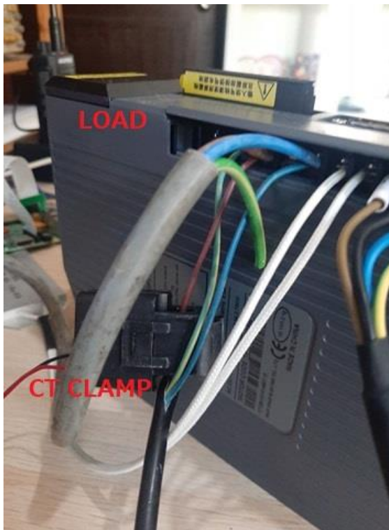
Fig. 3. Dummy load attached to the system to simulate a charging EV.
