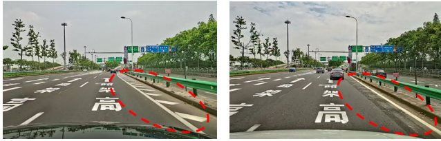
(a) The lane line before redrawn. (b) The lane line after redrawn.
