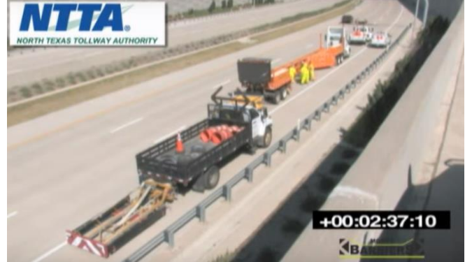
Fig. 1. Attenuator Truck Setup During Highway Work
