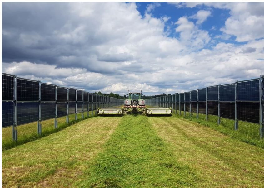
Figure 1: Vertically mounted agrivoltaic system with bifacial PV modules (Photo: Next2Sun GmbH).
