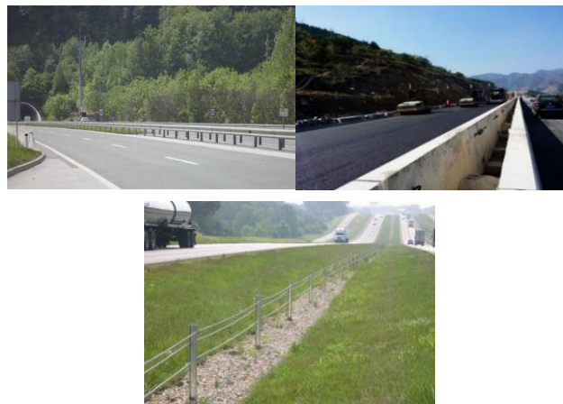
Fig.1. Several common highway barriers: (a) W-beam guardrail; (b) concrete barrier; (c) cable barrier
