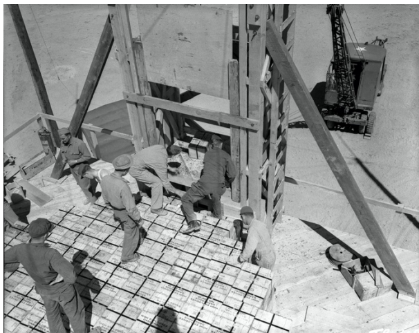
Figure 1. A photograph of the 100-ton test under construction.
