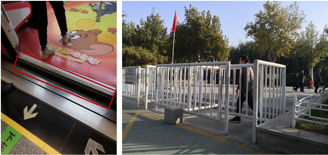
Fig. 3. (Left) Local subway system has a gap of over 100 mm between the train and the platform which can decrease the accessibility of the subway system to wheelchair users; (Right) the entrance gate of a park blocks wheelchair users.
