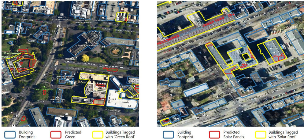
Figure 5: Geospatial engineering of the predicted result: tagging buildings with sustainable rooftops based on detected greenery and solar panels on them.
