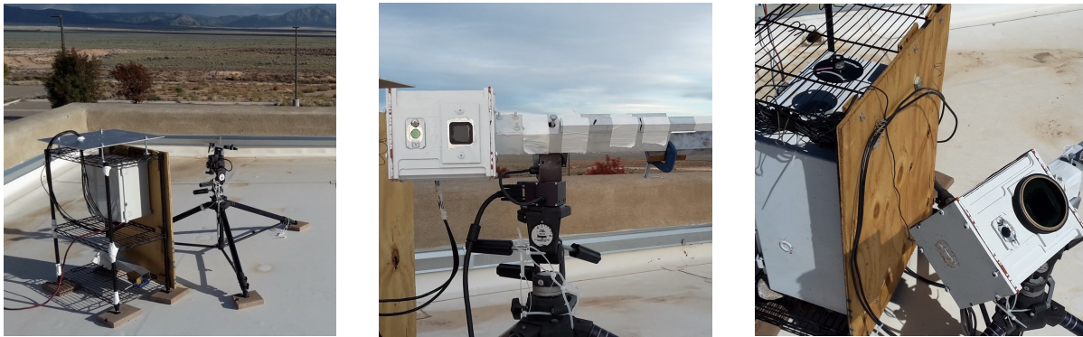
Figure 2: Tripod and junction box installed on the roof area of an UNM's facility. Solar tracker's servo motors mounted on the tripod, and screwed to a metallic structure which counterbalances the own enclosure's weight. The pyranometer is adjusted to a 3D printed support placed on top of the junction box's rack. Germanium and neutral density lenses for the IR and VI camera respectively, to filter the light beams and protect the cameras from weather hazards.
