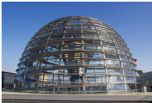
Fig. 2. The Reichstag Dome in Berlin, Germany. The metal features are both aesthetic and performative — they help resist radial and circumferential stresses.
