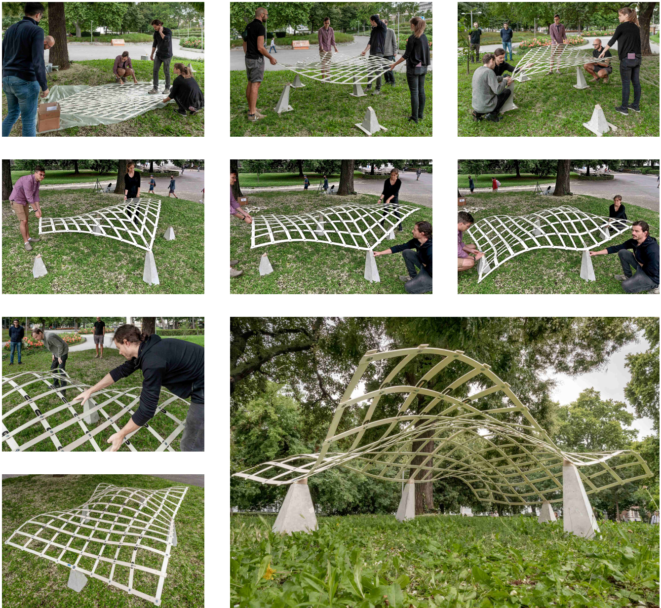
Figure 15: Several steps of the deployment of the EGG model and the deployed structure. The deployment process does not require a lot of force, and the curvature of the structure emerges naturally.
