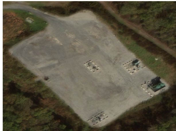
Fig. 3. This is an example of a fracking well during the production phase. The entire fracking process has been completed and the well will remain in this phase for 10-20 years. The only equipment on the pad are some holding tanks and the well heads. Image: DigitalGlobe, Inc.
