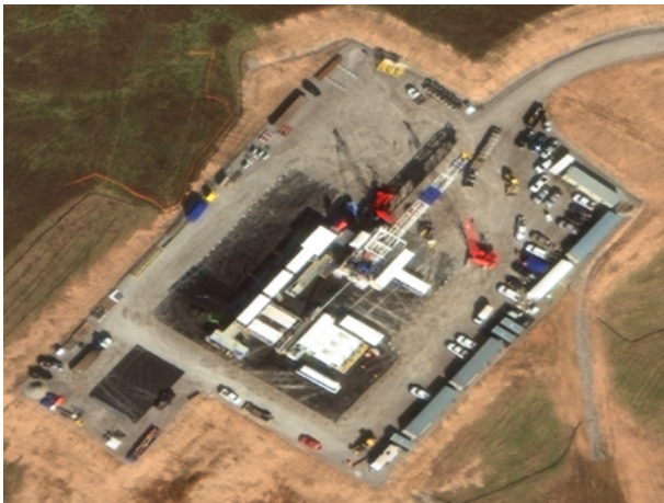
Fig. 2. This is an example of a fracking well during the drilling phase. A large drill tower can be seen in the center of the pad with multiple vehicles and other equipment surrounding. Image: DigitalGlobe, Inc.
