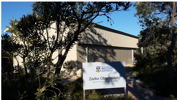
Fig. 1. External view of the Zadko Observatory.
