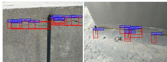
Fig. 1. Conflict between poor *mean Average Precision* (mAP) score and fine visual performance in crack detection. Demo images and their AP scores of the general objects (left) and cracks (right) are presented. According to the visual performance, the crack detector should not be such low scored (33.2).
