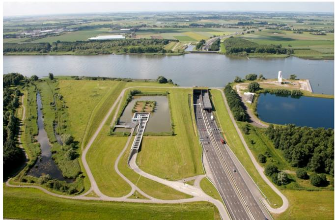
Figure 11: The Eerste Heinoord Tunnel (right) and the Tweede Heinoord Tunnel (left). Image from <https://beeldbank.rws.nl>, Rijkswaterstaat.
